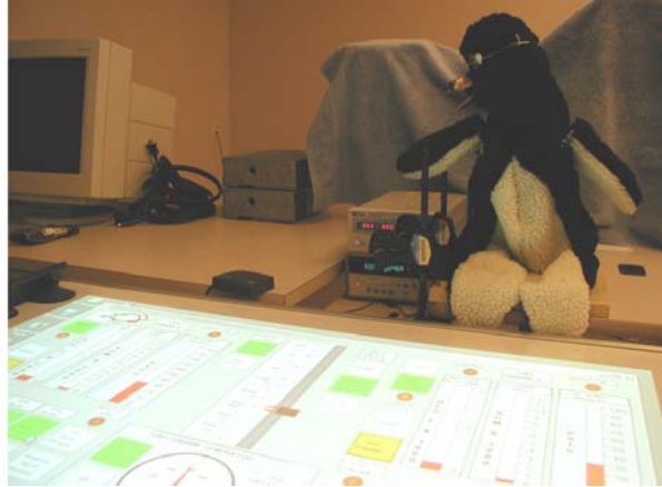
Figure 2. Mel pointing to the gas turbine control panel
